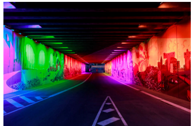
图 3 “资源回收”隧道 Fig.3 Recycle station tunnel
