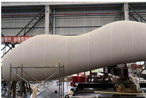
图 3 3D 打印桥梁装配现场 Fig.3 3D printed bridge assembly site
